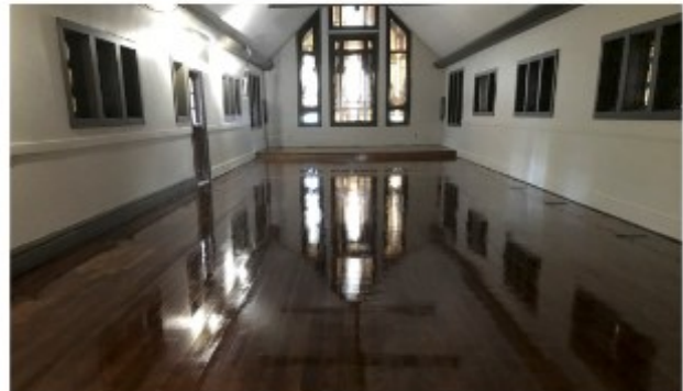
Nov 3 - floor stained and 1st coat of sealant
