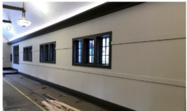
Nov 22 - picture rail installed
