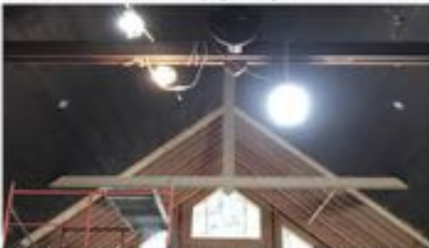
Sep 17 - new collar tie for camera & lights
