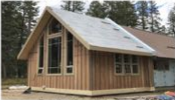
Sep 1 - board & batten finished on addition
