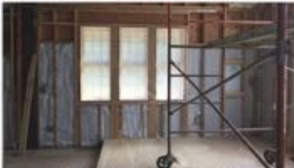
Sep 23 - insulation in the new walls
