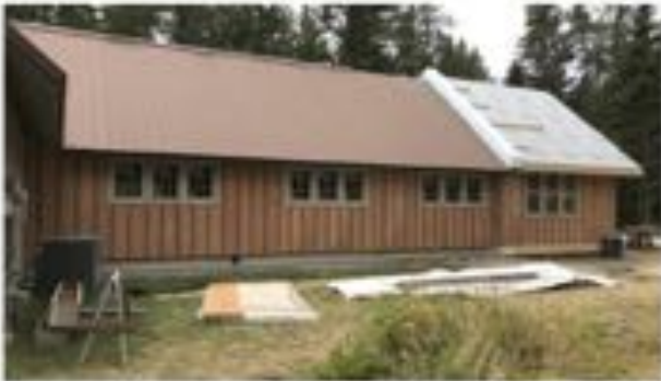
Aug 31 - board & batten finished north side
