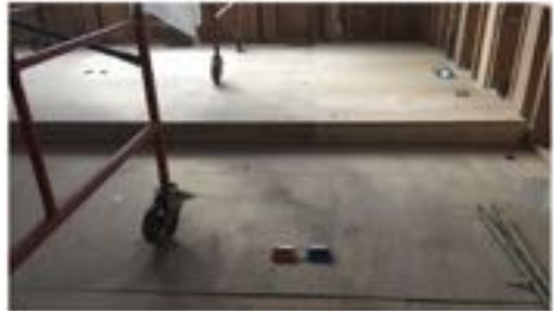
Sep 21 - platform completed & electrical for lectern
