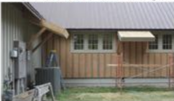
Sep 19 - overhangs to protect HVAC units
