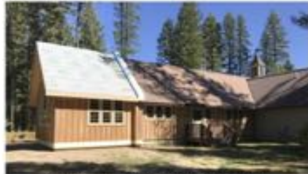
Sep 3 - board & batten all around
