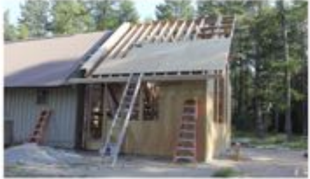
July 30 - plywood starts to go on the roof
