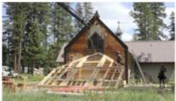
July 23 - back wall gets lifted into place
