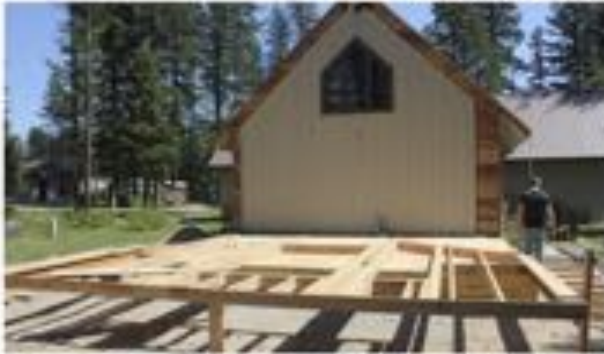
July 22 - Fr Charlie checking out the walls
