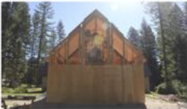
July 24 - rafters in place and some plywood
