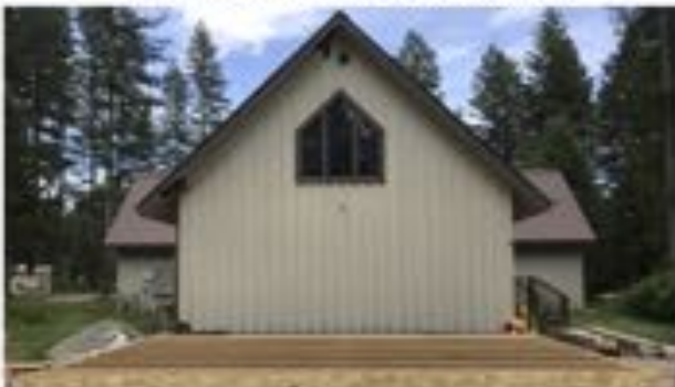
July 15 - floor joists down
