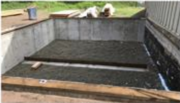
July 7 - preparing for floor joists
