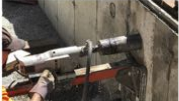
July 9 - concrete drilled for core testing
