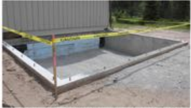
June 12 - gravel in what will be crawl space
