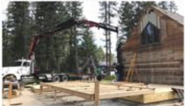
July 23 - north side frame is set
