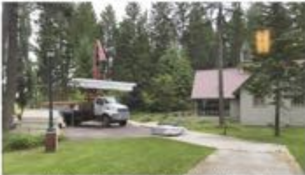
July 1 - flooring materials delivered
