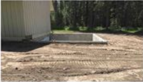
June 1 - foundation back filled
