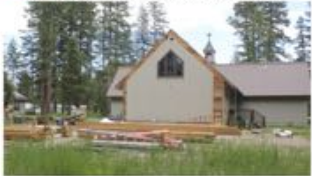
July 16 - prepping for steel moment frames
