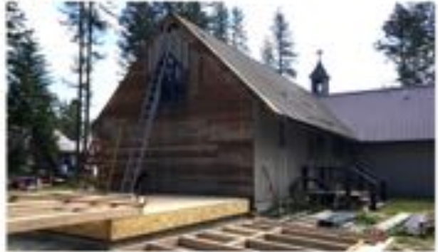
July 23 - almost ready for the moment frame
