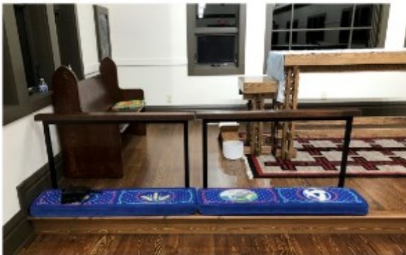
Jan 21 - altar rail redone - new steel tubing and original 100 year old wood
