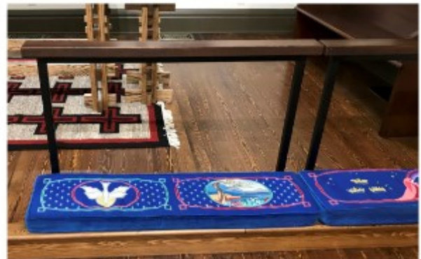
Jan 21 - altar rail redone - new steel tubing and original 100 year old wood
