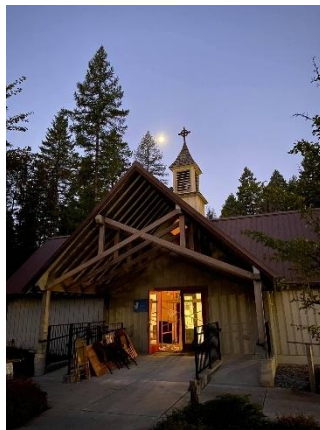
Figure 10: Remodeling the Sanctuary
